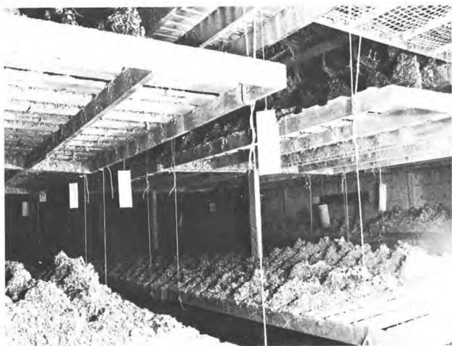
Plate 5.4. The pit beneath a battery hen house where droppings accumulate.
