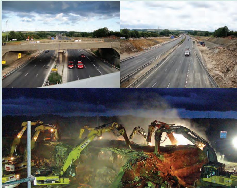
Top left and right: Saturday night and Sunday morning on the M1. Bottom: teams working for the Highways Agency attack the structure overnight
