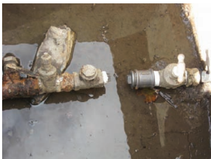
Figure 1.6 Removal of Cross-connection Between Public and Private Water Supply
