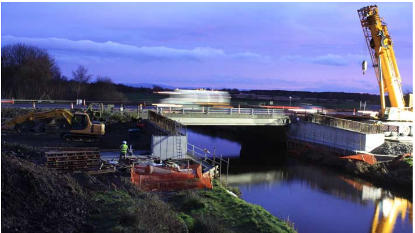
Faughan Bridge on the A2 Broadbridge scheme
