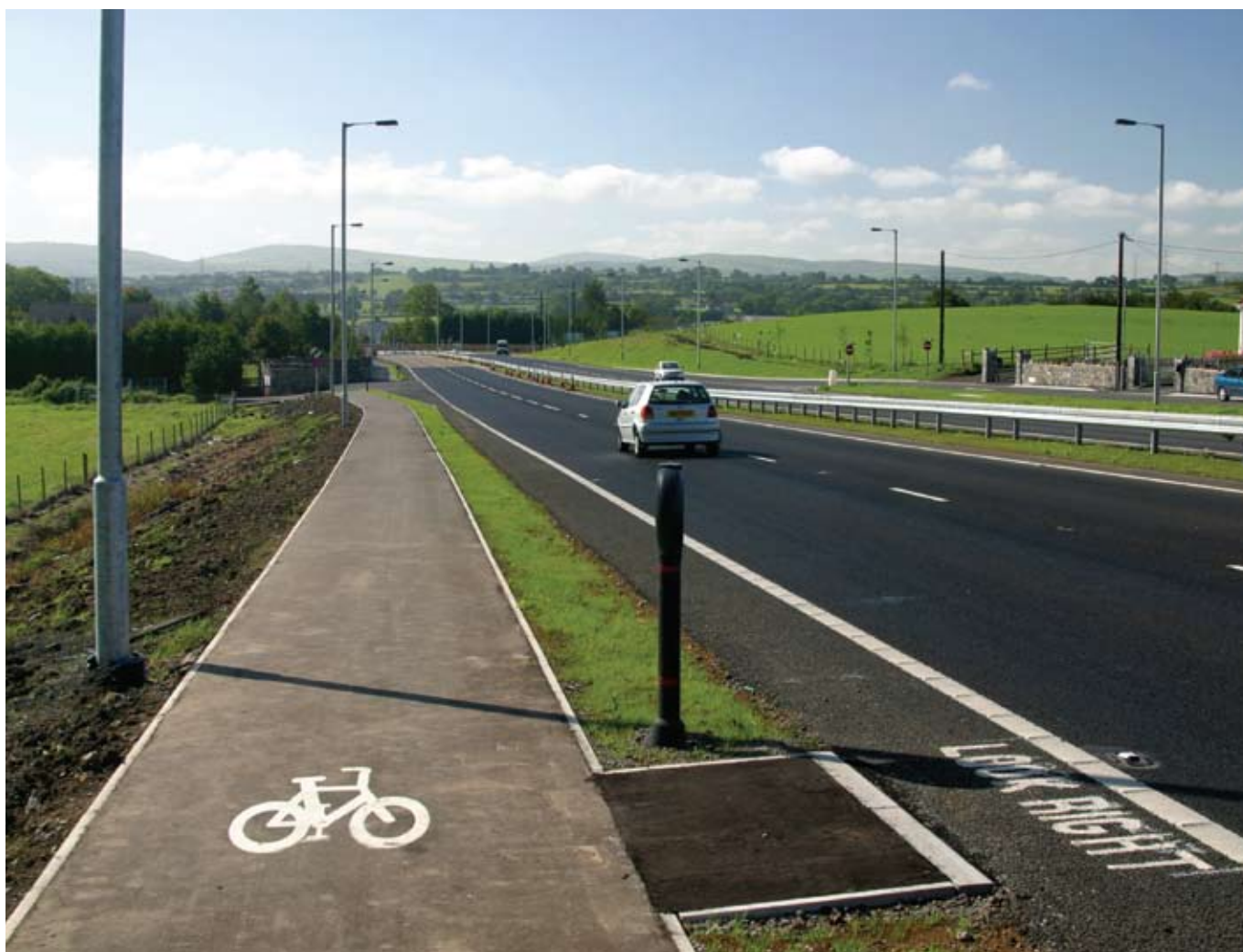
A8 Doagh Road to Coleman's Corner dualling.
