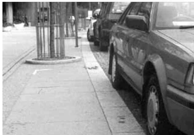
Figure 6.5: Use of surfaces, textures and planting to define kerb free level access parking bays (Source: Planning and access for disabled people: a good practice guide 2003 )
