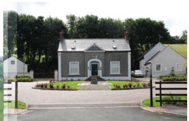
Fincarn Cottage, restored with NIEA grant assistance
