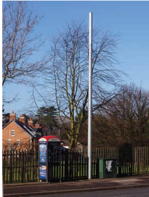
An example of a slim-line monopole. A simple well-proportioned installation.
