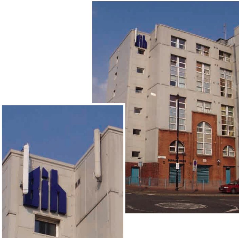
Two pieces of telecommunication equipment. Unfortunately only one mast is painted to minimise visual impact.
