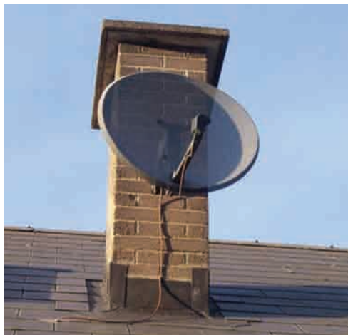
Chimney Mounted Satellite dish.
