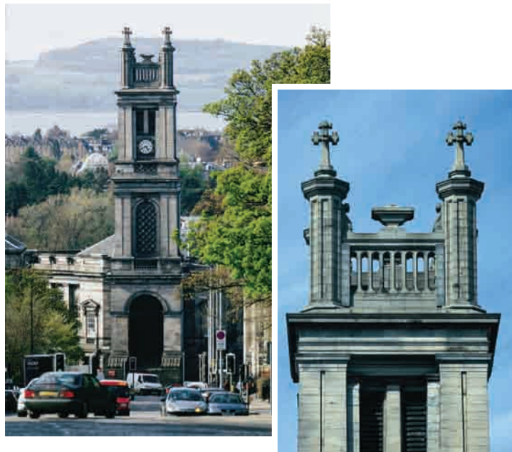
St Stephen's Church in Edinburgh has eight mobile telecommunications antennas mounted behind fibreglass panels painted to match the stonework at the top of the tower and a cabin inside the tower itself.
