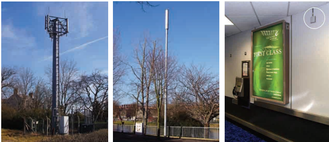
Examples of Macrocell, Microcell and Picocell equipment.
