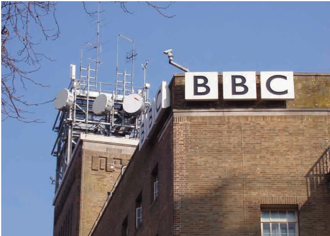
Microwave dish antennas located on top of a broadcasting building in Belfast City Centre.
