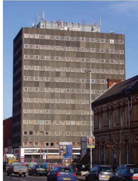
Telecommunications equipment installed on top of a large office block in Belfast.
