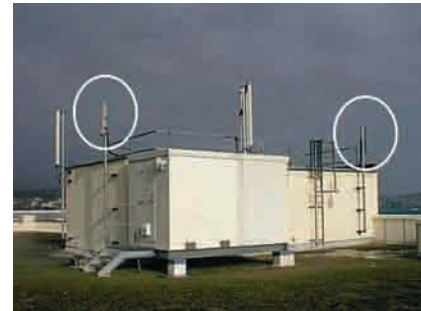
Second and third Generation equipment on a rooftop site. The 3G equipment is highlighted.
