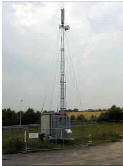
An example of a temporary Telecommunications Mast.
