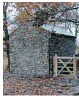
A National Park stone cabin to house equipment
