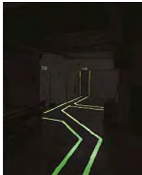
Figure 56: A way-guidance system
