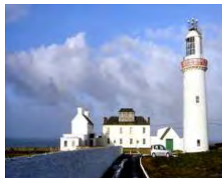
Loop Head Lightkeepers House, Co. Clare
