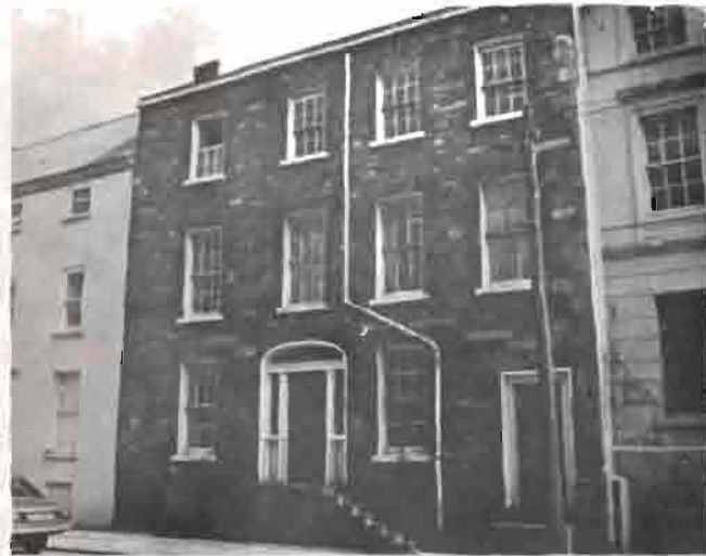
The balance of fenestration and vertical window proportions essential to the character of the Conservation Area are illustrated in this Georgian terrace house.
