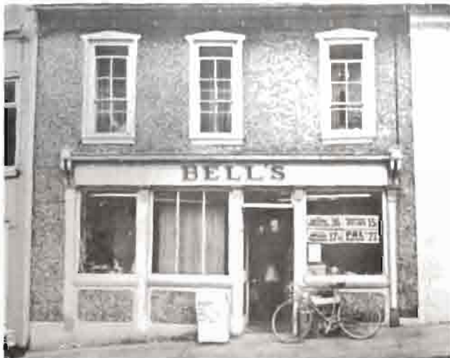
The importance of good signs is illustrated in these two shopfronts. Compare them also with examples of shopfronts at the rear of the booklet.
