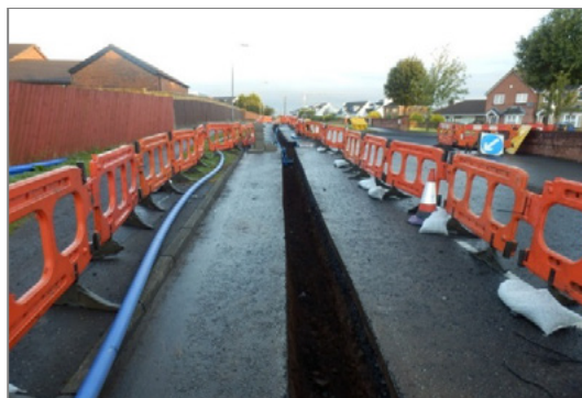
Figure 2.8: New Mains Installation
