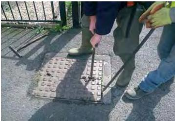
The manhole lifters should fit snugly and securely into lifting eyes. The manual lifters should be around 500mm to 600mm long and have anti-slip ends as shown below.
