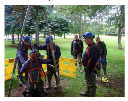
There is a weight limit for staff involved in underground working which has been imposed due to the Safe Working Load (SWL) of the winch. This weight limit takes account of the necessary equipment UG workers may carry with them.
