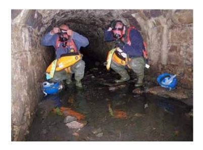
HARD HATS. The most suitable hard hat for use in underground work has a shorter peak and a head torch is worn on top of the hard hat as shown below.
