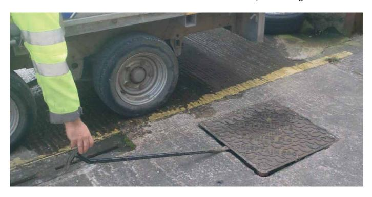
Mechanical lifters are also available for covers which are difficult to free. Proteous mechanical lifters are available for use if required (see photograph below). They are most useful when the area surrounding the manhole has blacktop or a surrounding hard surface.
