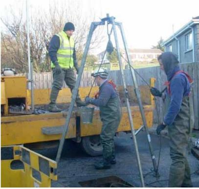
The tripod is constructed from aluminium and is designed for rapid set up. The tripod is adjustable in height from 1.4 to 2.42m and the legs can be set up with a diameter range from 0.99 to 1.55m. The length of the wire rope in the winch is approximately 4.5m long. The winch has a gearing mechanism which allows controlled descent of both persons and materials. The winch is also used for the removal of debris in buckets.
