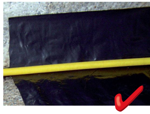
Photo 9 – Protecting silage pit wall-floor joints
