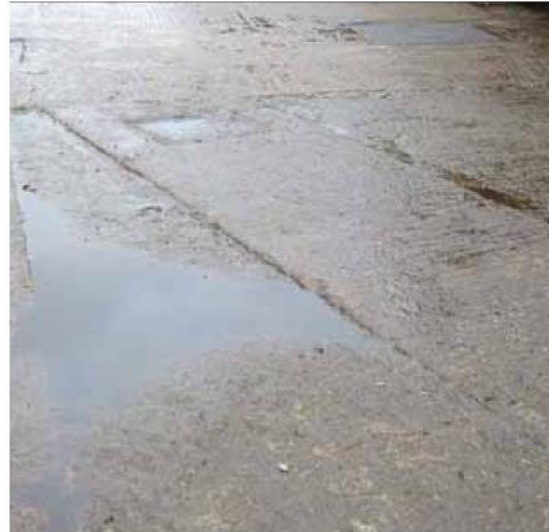
Photo 26 – Run-off from a frequently used roaming yard is slurry.
