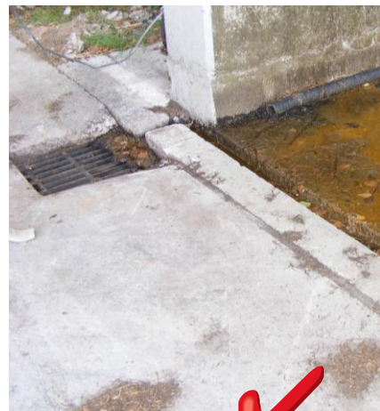
Photo 13 – Silage clamp with well maintained channels draining to effluent tank
