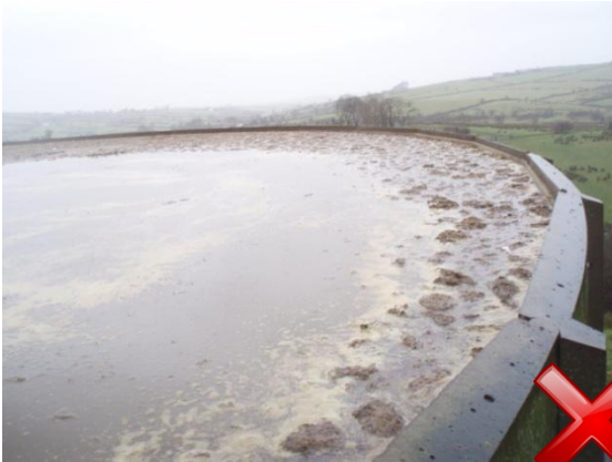
Photo 10 - Freeboard on above ground slurry tank not being maintained
