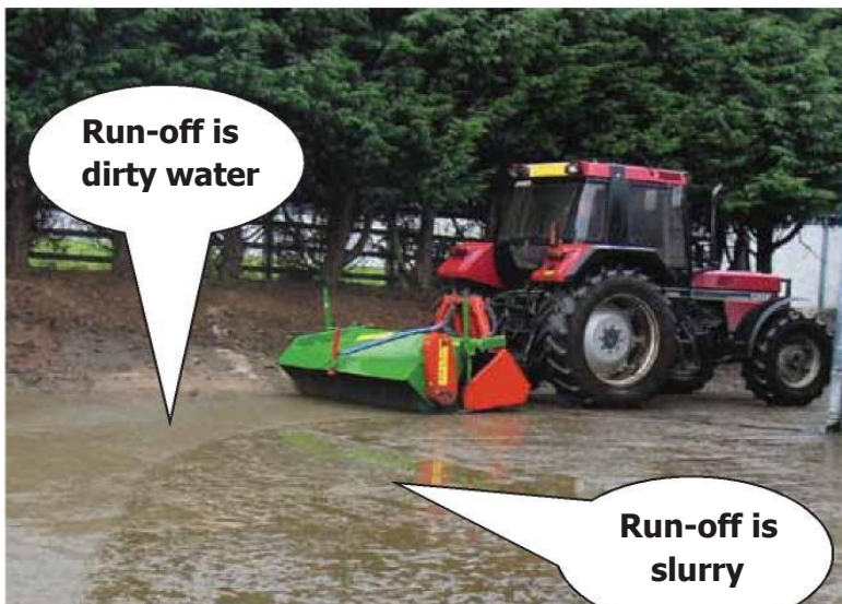
Photo 27 - The removal of slurry from yard areas will reduce the requirement to store slurry.
