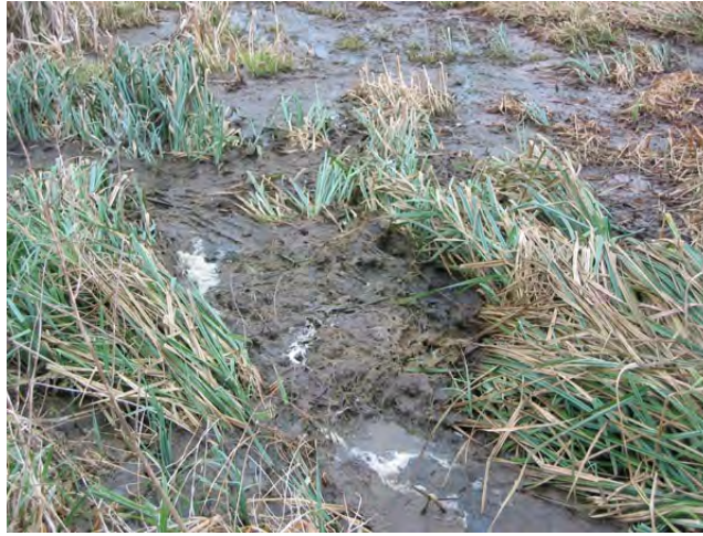
Figure 15: Sediment accumulation in the initial cell of a CFW.
