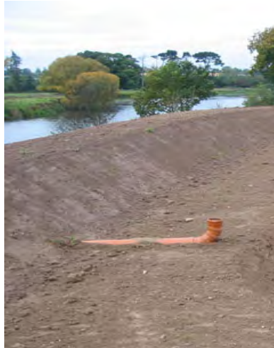
Figure 8. Outlet pipe with an adjustable bend.
