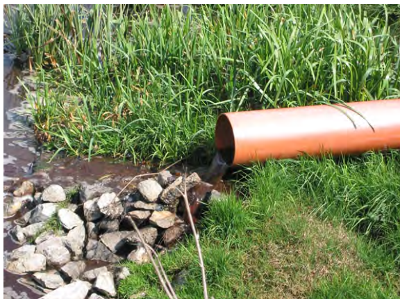
Figure 7: Inlet pipe to CFW cell
