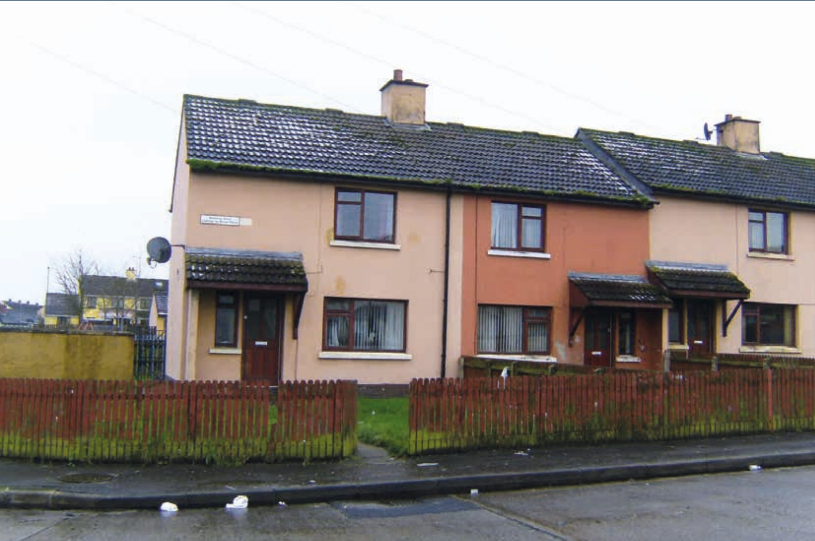
Houses at Rinmore before refurbishment: photo courtesy of DSD
