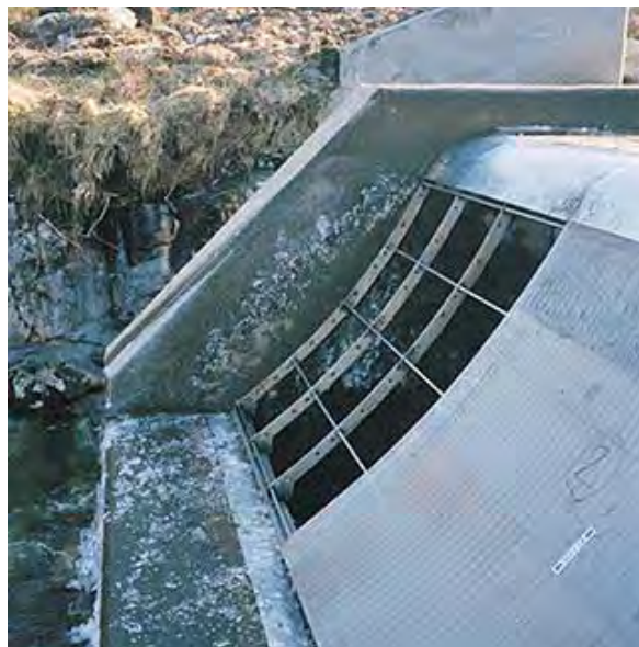
Figure 4.5: Example of a Screen A Coanda installation (Dulas Hydro).
