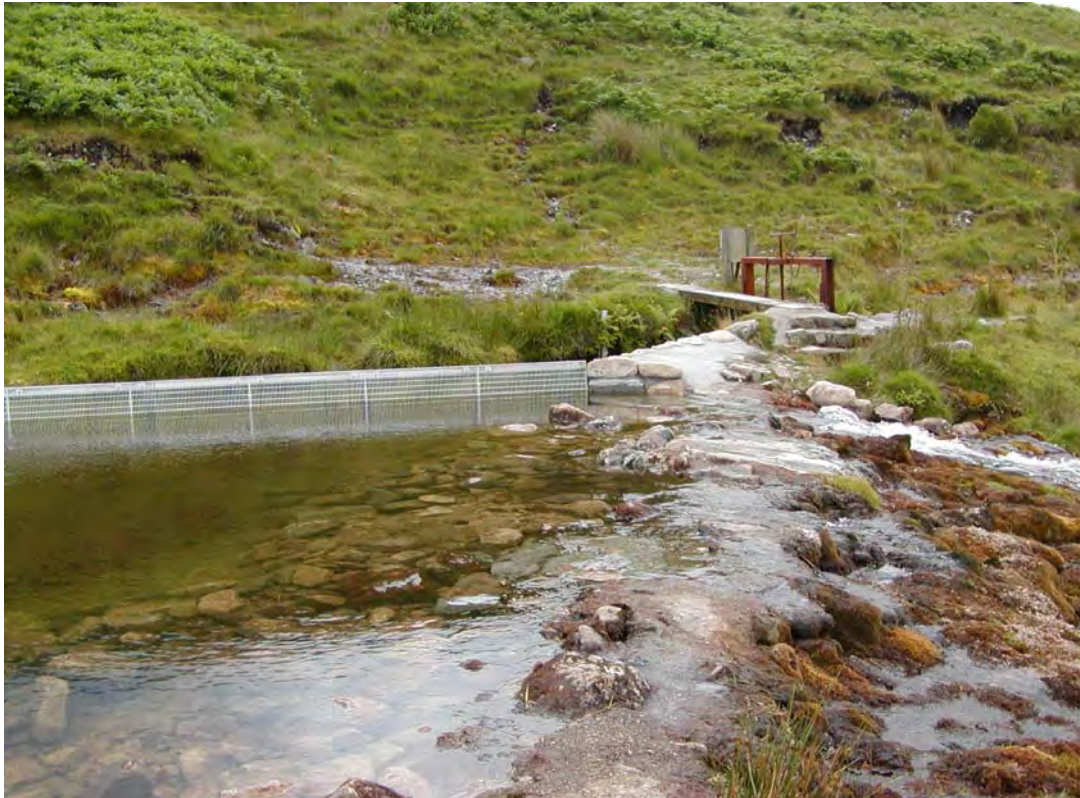
Figure 4.2: Fixed panel screen installed in 2003 on the River Plym, Devon. It protects the entrance to an industrial supply offtake.
