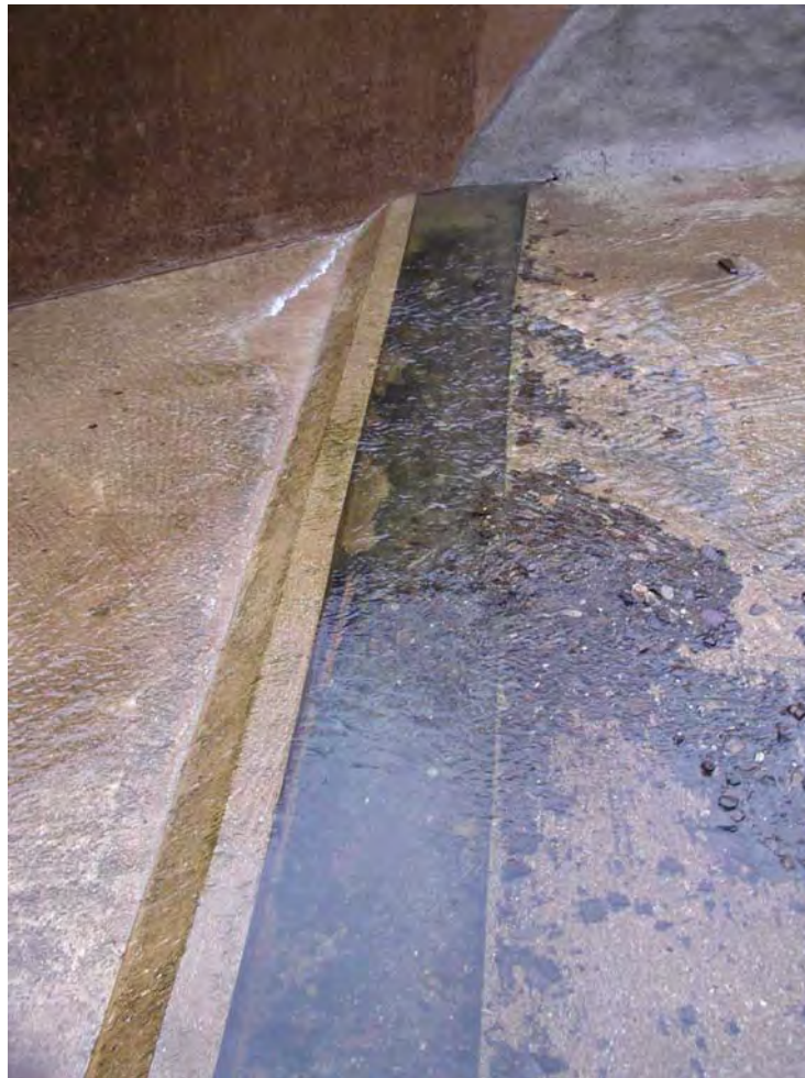
Figure 7.3: The eel bypass trough at the Backbarrow hydropower scheme on the River Leven, Cumbria (Spiby, 2004). The trough is formed along a diagonal in the floor of the headrace canal, with a submerged bywash at its downstream end. The flow in this picture is from right to left.
