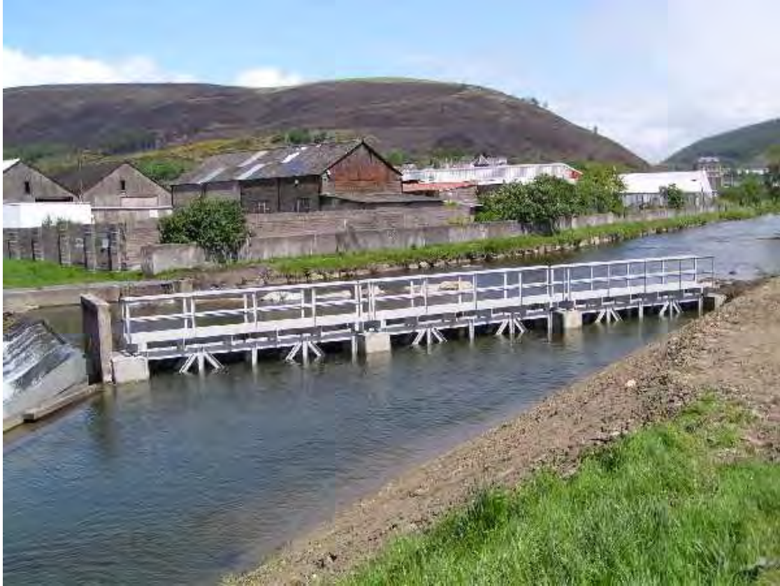
Figure 4.1: Fixed panel screen installed in 2003 on the River Afan, Port Talbot, to prevent salmonid smolts from entering the docks' feeder.
