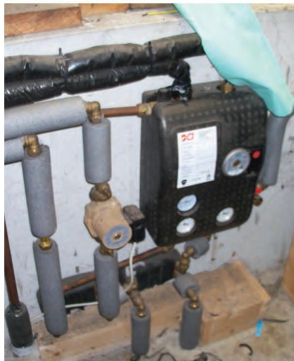
Solar controls and heat distribution system
