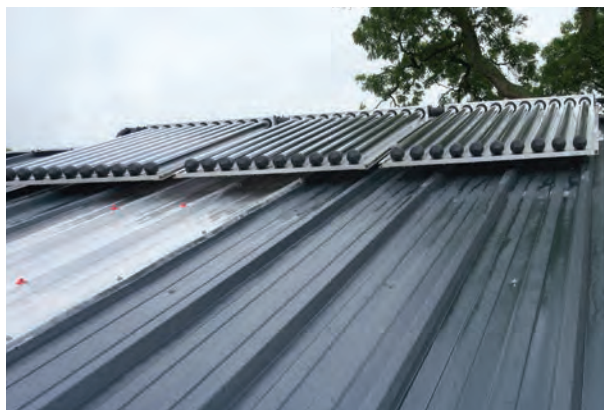
Solar tubes mounted on the dairy roof
