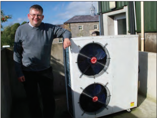
CREAM Dairy Air Source Heat Pump Installation
