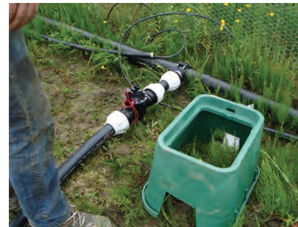
Automated valve construction
