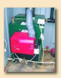
inefficient oil boiler. The new boiler works at above 90% efficiency compared to the 65% level of the original boiler.
