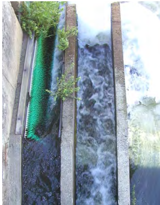
Figure 6.2. Detail of eel pass at Moulin a Pigné
