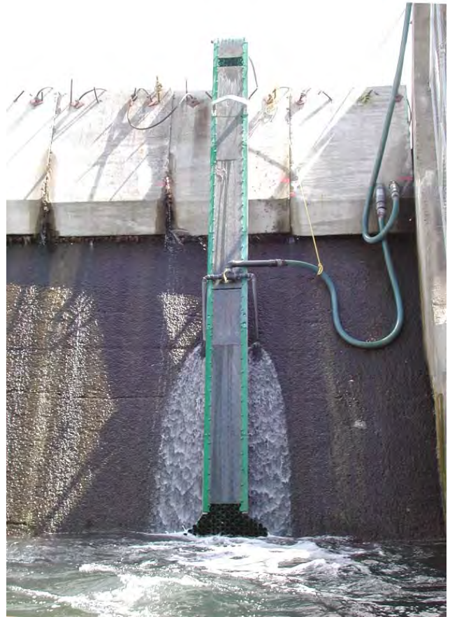
Figure 6.7. Eel pass at Chambly Dam. Note the breakwater blocks on the dam crest, and the gravity-fed attraction water being discharged from the two pipes part way down the dam face. Photo D. Desrochers.
