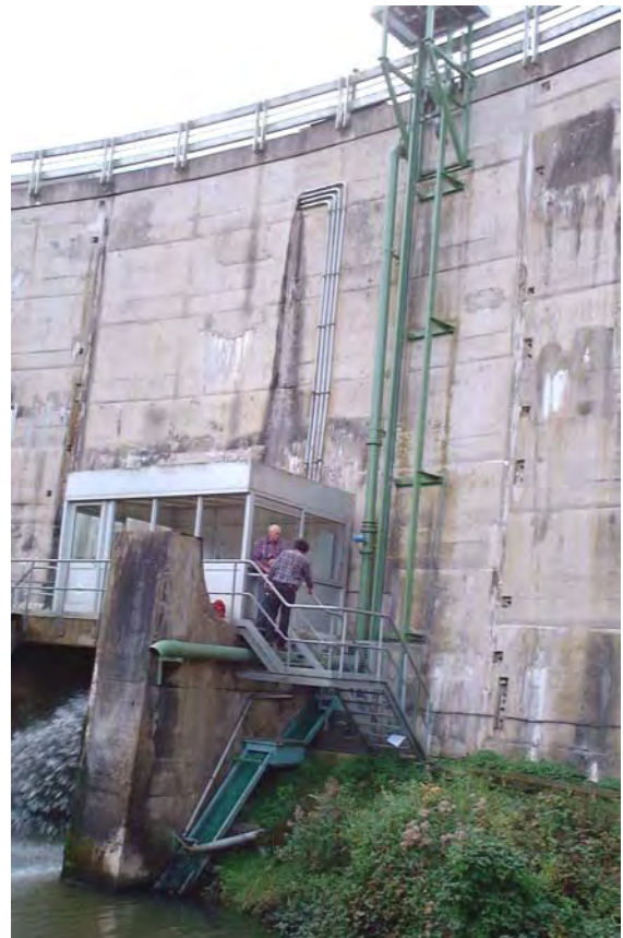
Figure 6.12. The Ville Hatte Dam eel lift. The substrate ramps can be seen below the platform.
