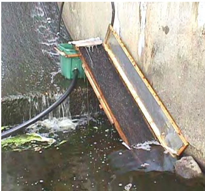
Figure 6.16. A “portable passage” being operated at Benton Falls Dam in Maine. The cover is lifted to show the Enkamat substrate. Photograph G. Wippelhauser.
