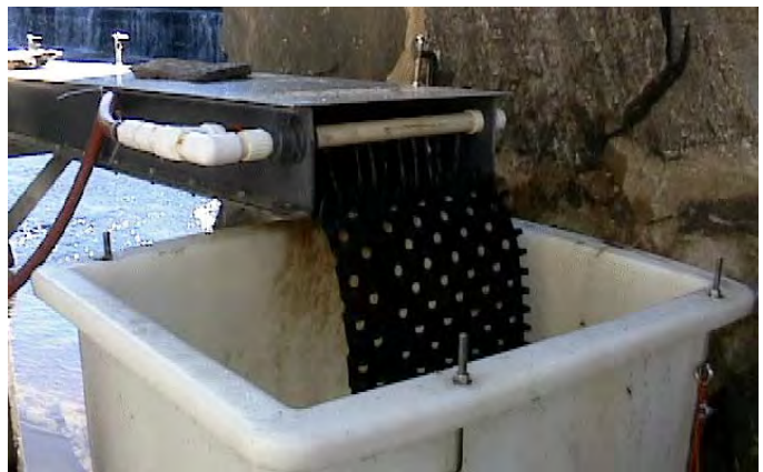
Figure 6.11. Akwadrain substrate extending beyond the top of the ramp at Greenville Dam eel pass. Photograph Alex Haro.
