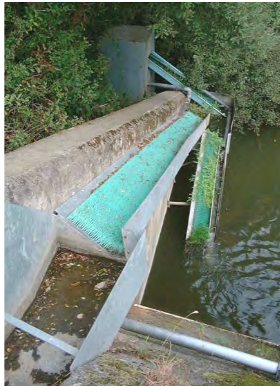
Figure 6.3. Upstream pass and pass-trap at Pont-es-Omnès
