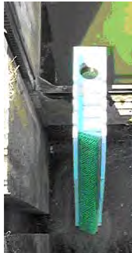
Figure 6.15. “Fish-Pass” prefabricated sluice-gate pass.
