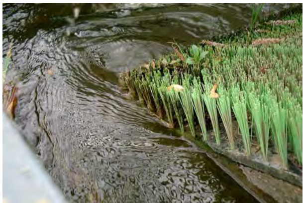
Figure 6.5. Flow to the baffle pass cutting across the top of the eel pass, Chadbury. The flow down the pass is from left to right.
