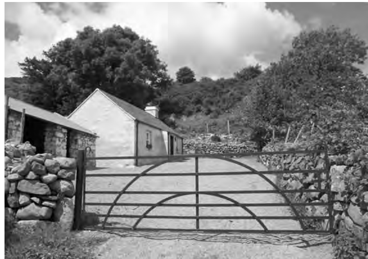
The newly restored Rock Cottage photo courtesy of NIHE
