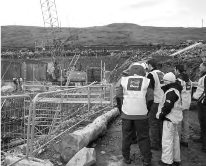
Visit by Bangor University (Wales) to Fofany water treatment project.
