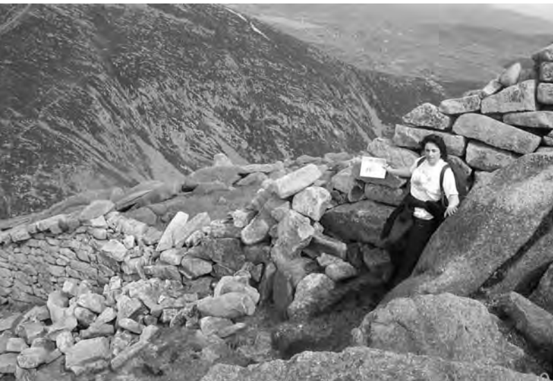
Inspection of the Mourne wall carried out by Mourne Conservation Volunteers
