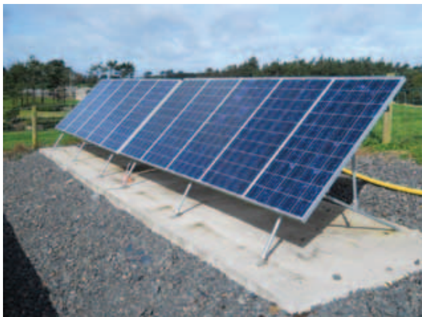
Figure 1. Solar PV panels fixed together on a frame. Each panel has a dimension of 163cm x 81cm
