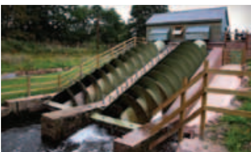
Two Archimedes screw water Turbines installed side by side, Devon England
