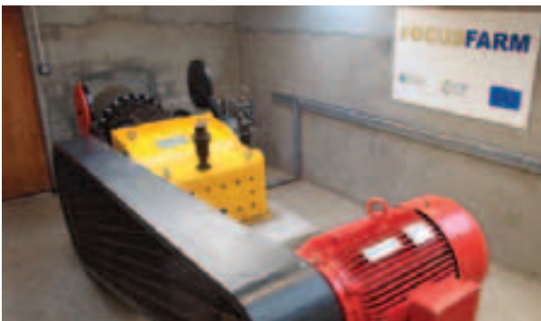
A Crossflow Turbine installed at the McCambridge Focus Farm just outside Ballycastle
