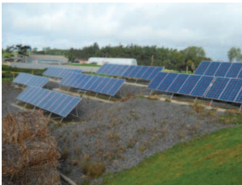
Figure 2. An array of seven stand-alone PV modules set on a southern facing slope at AFBI Hillsborough. Note the angle of the panels – some are set at 43° and some at 51° off vertical
