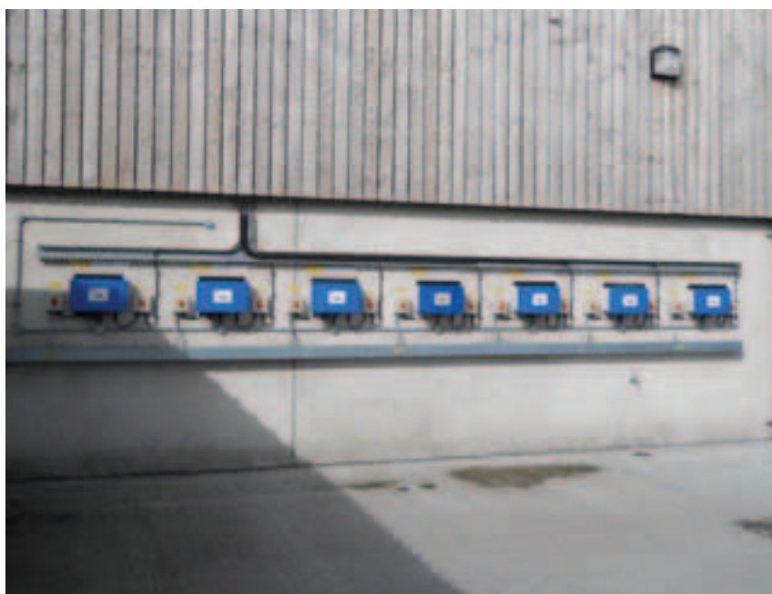
Figure 3. The seven Inverters for the AFBI Hillsborough PV array. Each module is connected to a single inverter and the current then transformed to AC is passed directly into the electrical network
