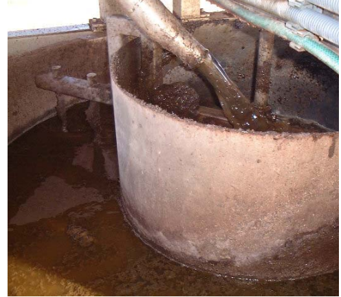
(b) Addition of polymer to enhance solids removal
