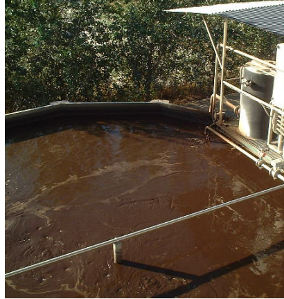
(a) Reactor tank for removal of slurry N
