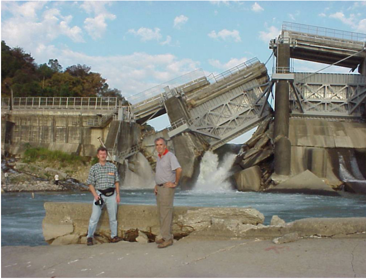
Figure 3.51 Instability of concrete dam (Natural Resources Canada).
