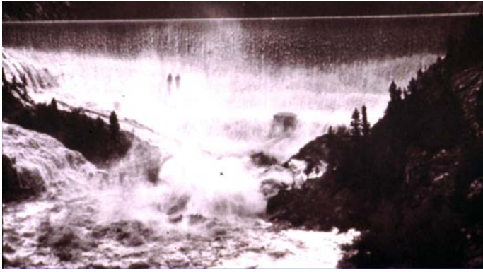
Figure 3.55 Structural failure of concrete dam (England, 2009).
