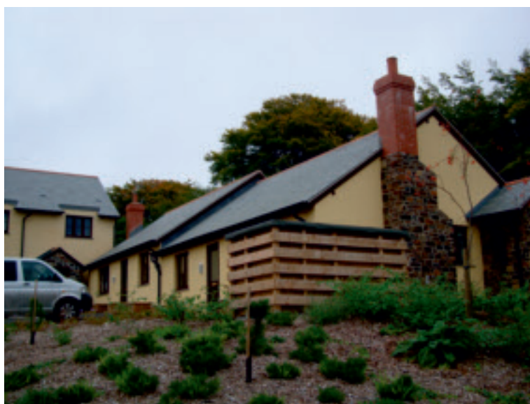
A new development of affordable housing in Exford, Exmoor National Park, constructed using 'hemcrete', heated with locally sourced woodfuel.
