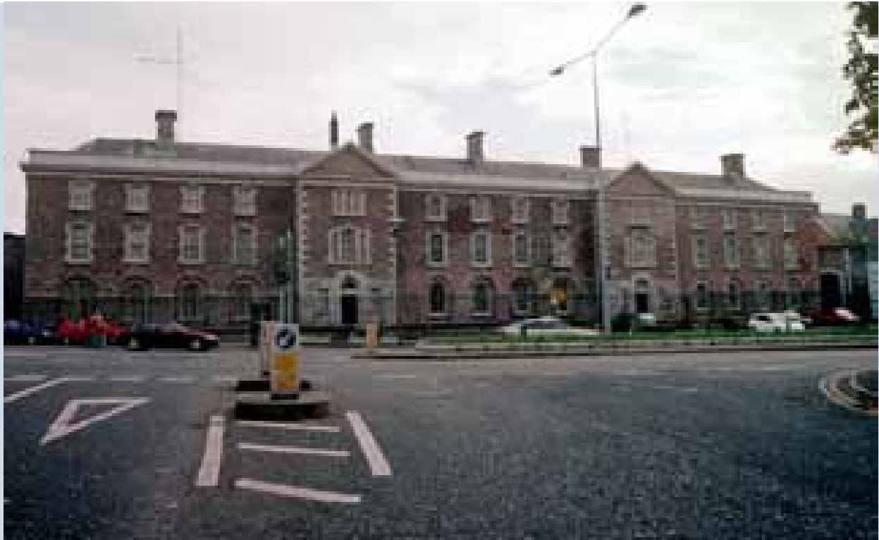
Figure 12: Armagh Gaol – formerly owned by the Northern Ireland Office
