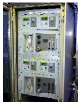
Diagram 17: Controlled atmosphere killing unit gas mixing panel
