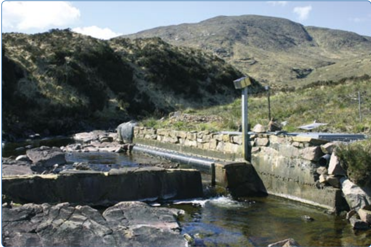
High head run of river intake with constructed head weir.
