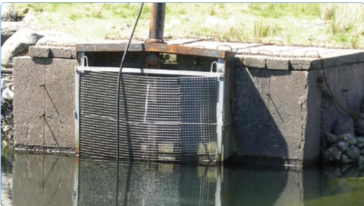
High head run-of-river intake screen.
