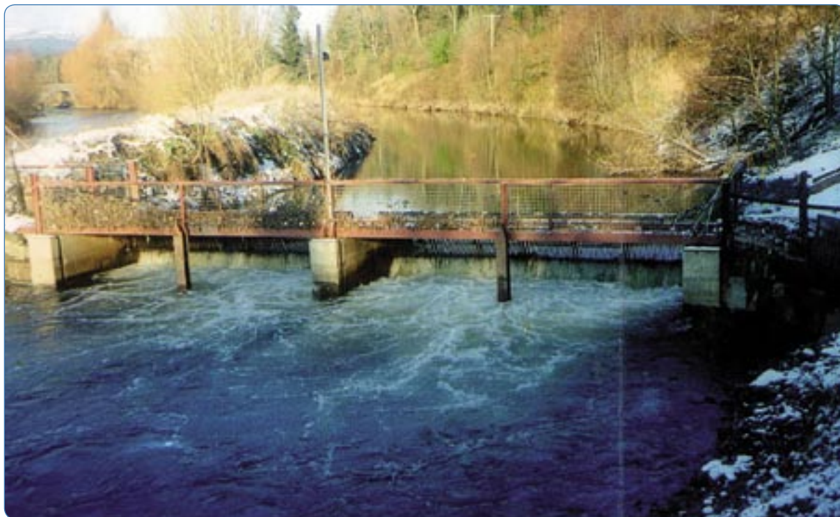
Fixed screen installation at point of return of tailrace flow to main river. This screen will prevent the entry of upstream migrating salmon entering the tailrace.
