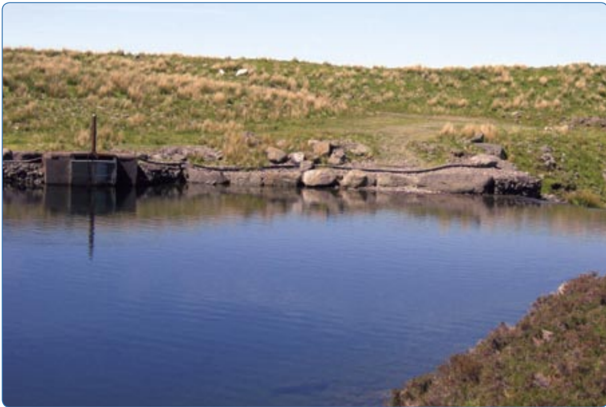
Turbine intake on a high head lake impoundment.
