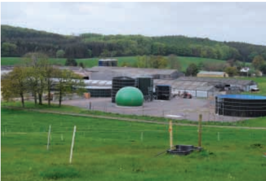
Anaerobic Digestion plant at AFBI Hillsborough
