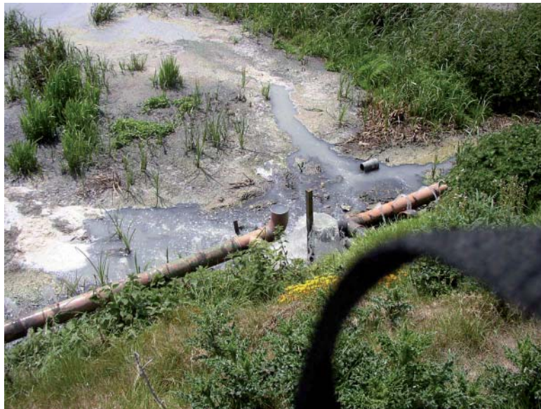
Figure 10 Vertical Flow inlet at Kilmeaden surface flow Constructed Wetland
